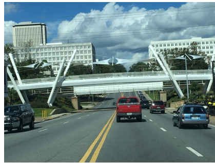
Figure 6a. View of footbridge driving from the south toward Tallahassee’s Downtown with railroad bridge in the background.
