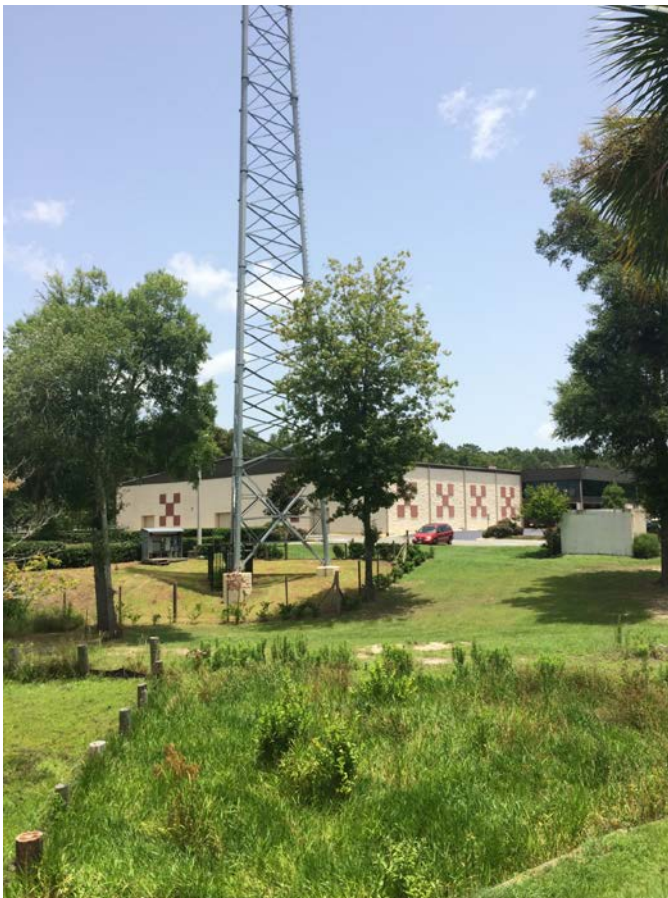
Figure 3. D&F Communications tower location.
