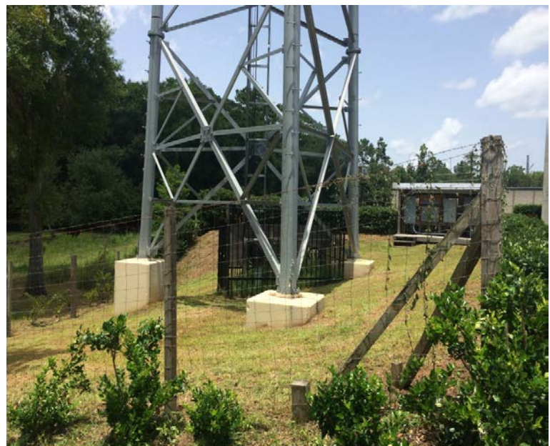
Figure 4. Base of D&F Communications wireless tower.
