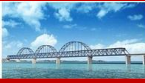
Yellow River Bridge of Beijing-Shanghai High-Speed Rail
